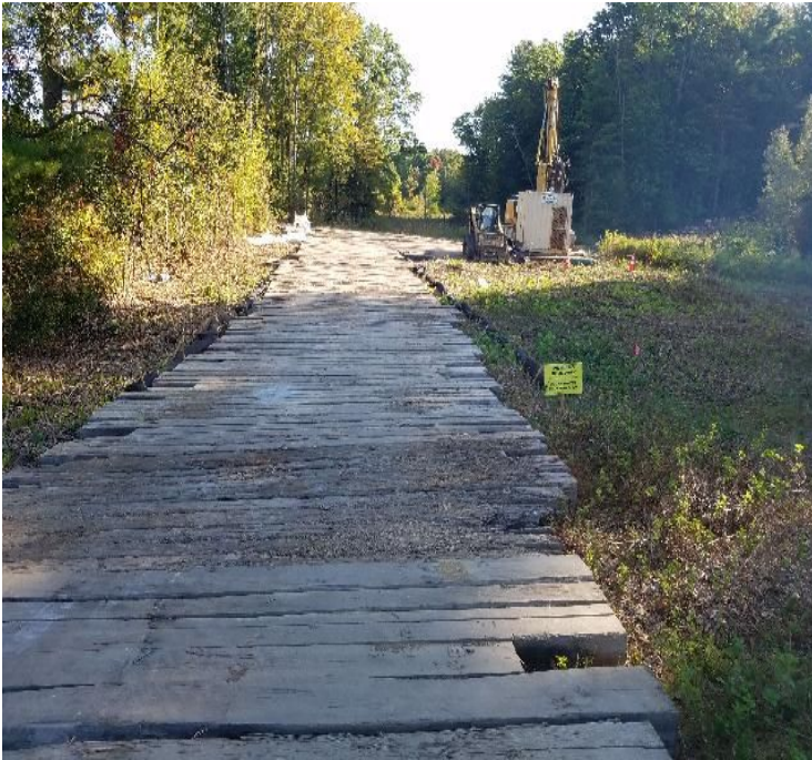
Fig 5: Access to Str. 112. Viewing north. (9-24-19).
