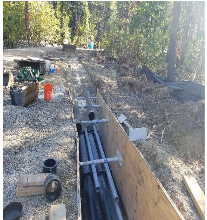
Fig 16: Continued install of pipe next to Flynn pit. Viewing east. (9-25-19).
