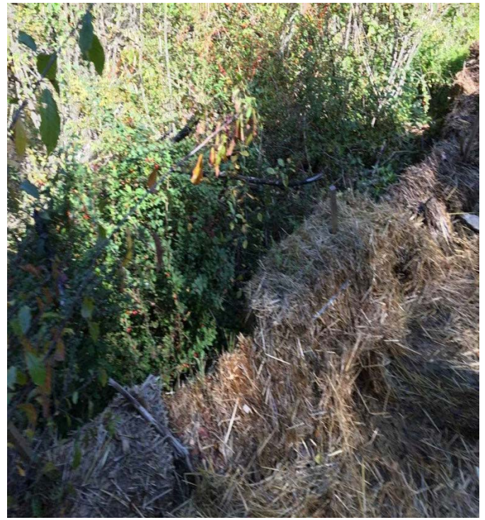
Fig 18: Siltation controls along Oyster have been replaced. Viewing north. (9-25-19).
