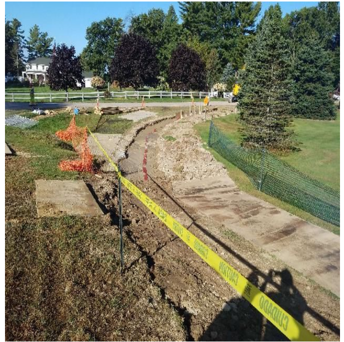
Fig 14: Backfilling and restoring trench area along Gundalow Landing. Viewing west. (9-25-19).
