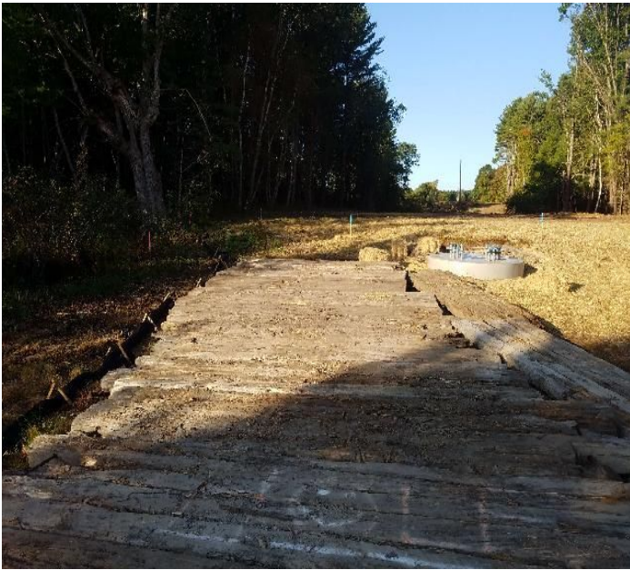
Fig 1: Str. 106. Viewing west. (9-24-19).
