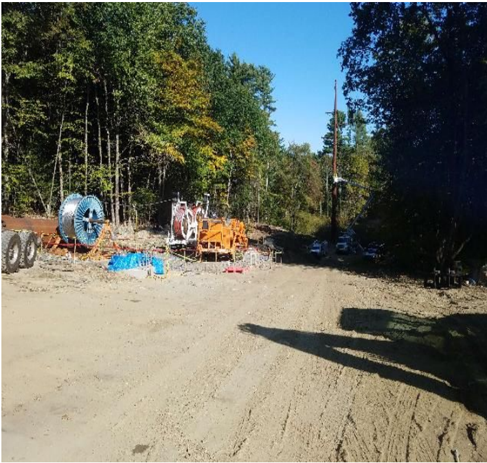
Fig 9: Pulling wire at Str. 28. Viewing north. (9-24-19).
