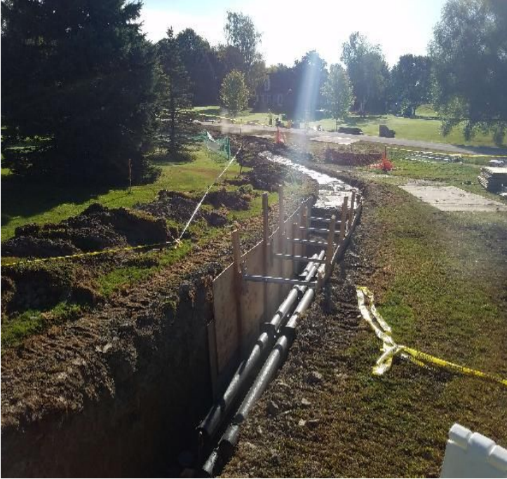
Fig 13: McCourt continues to fuse pipe along Gundalow Landing. Viewing west. (9-25-19).
