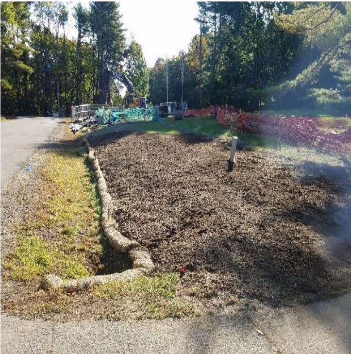
Fig 15: Restoration and seeded trench area along Gundalow Landing. Viewing east. (9-25-19).
