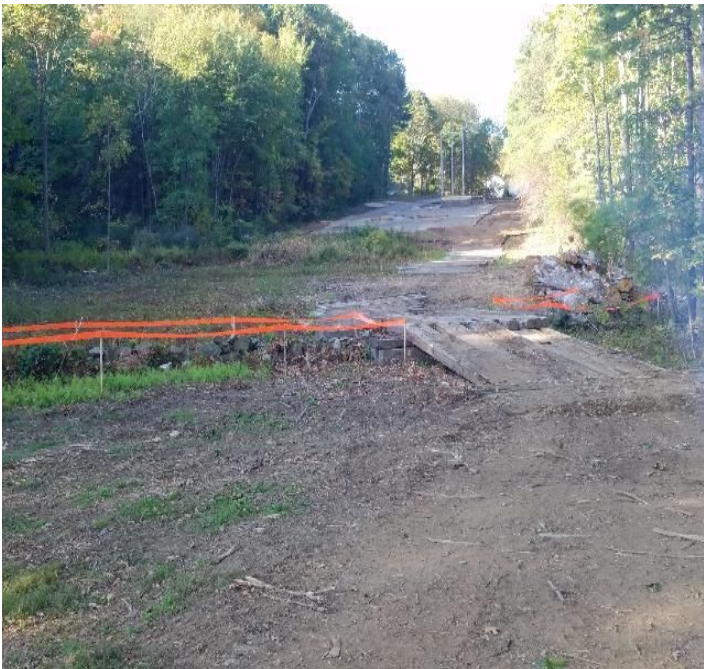
Fig 3: Access to Str. 107. Viewing southwest. (9-24-19).
