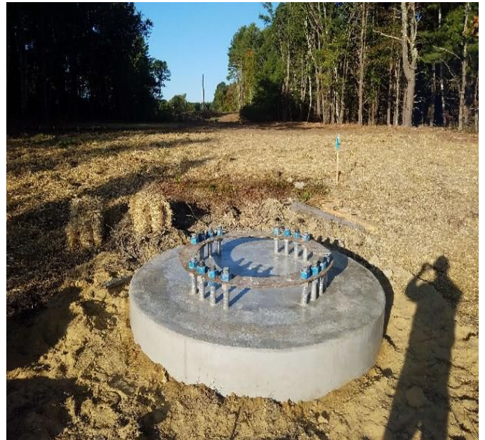
Fig 2: Exposed soils covered around Str. 106 foundation. Viewing west. (9-24-19)
